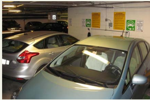
The underground parking garage that services the CRC is home to several electric vehicle charging stations.
